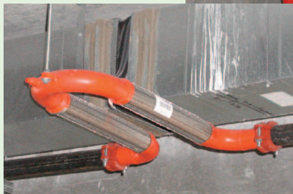
Thirty Fireloop expansion loops, installed parallel to the ceiling, were placed at the building's separation joint in mains and branch lines throughout the building.
