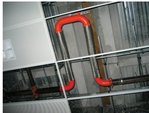
Fireloops permitted tighter piping runs and fit close to walls and ceilings.
